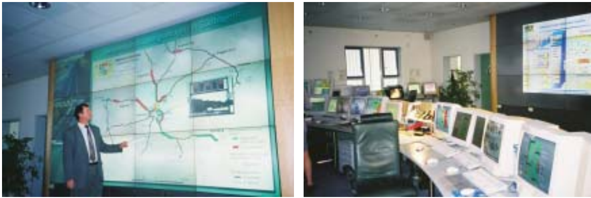
Figure 27. VRZ traffic management center.
