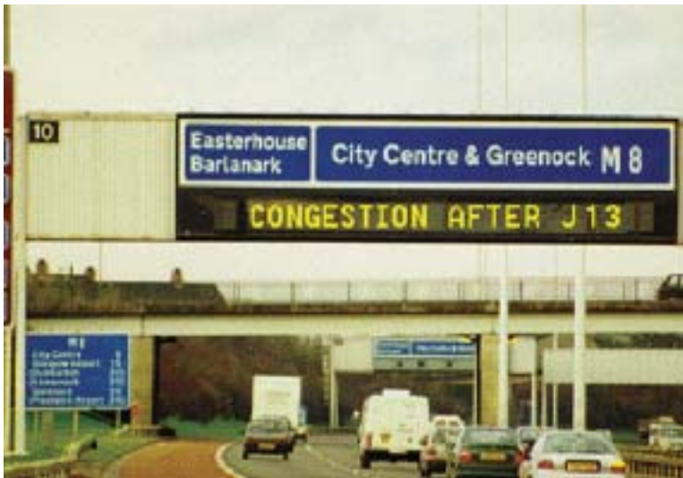
Figure 51. Message sign in Glasgow.
